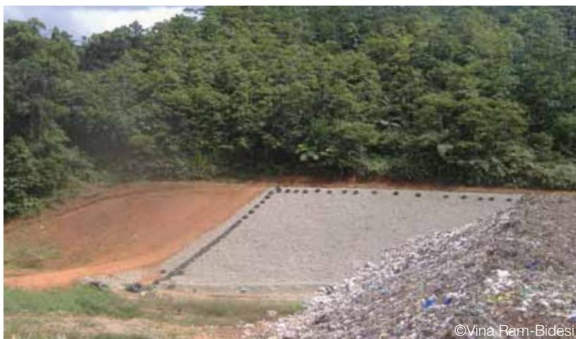
A new 'state of art' landfill in Naboro which replaced the original Suva dumpsite in a coastal mangrove area.
