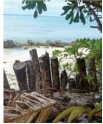
Figure 202 Collapsed Concrete cube Seawall at Nanumaga. Figure 203 Collapsed Concrete cube revetment at Funafuti. Figure 204 Collapsed Gabion basket wall and Tree Trunk wall at Nukulaelae. (Source: Fig.203: Tuvalu NBSAP)
