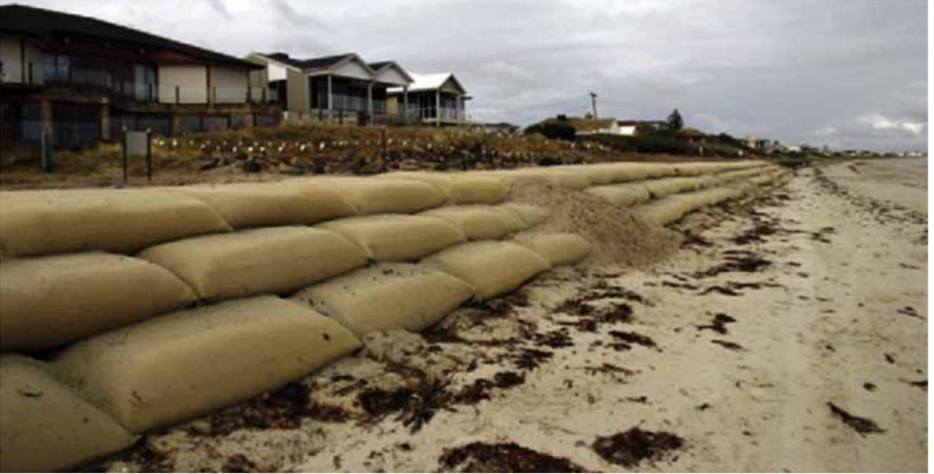
Figure 23: Geotextile Sand-filled Container (Elcorock) Revetment Example
