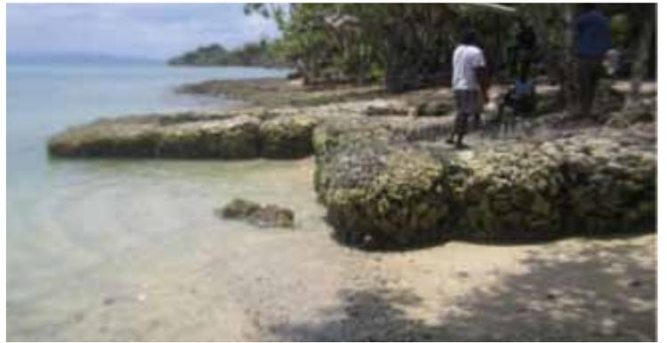
Figure 175 Gabion basket at Worasiviu.
