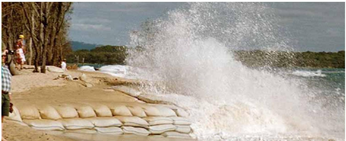
Figure 22: Geotextile Sand-filled Container (Elcorock) Seawall Example
