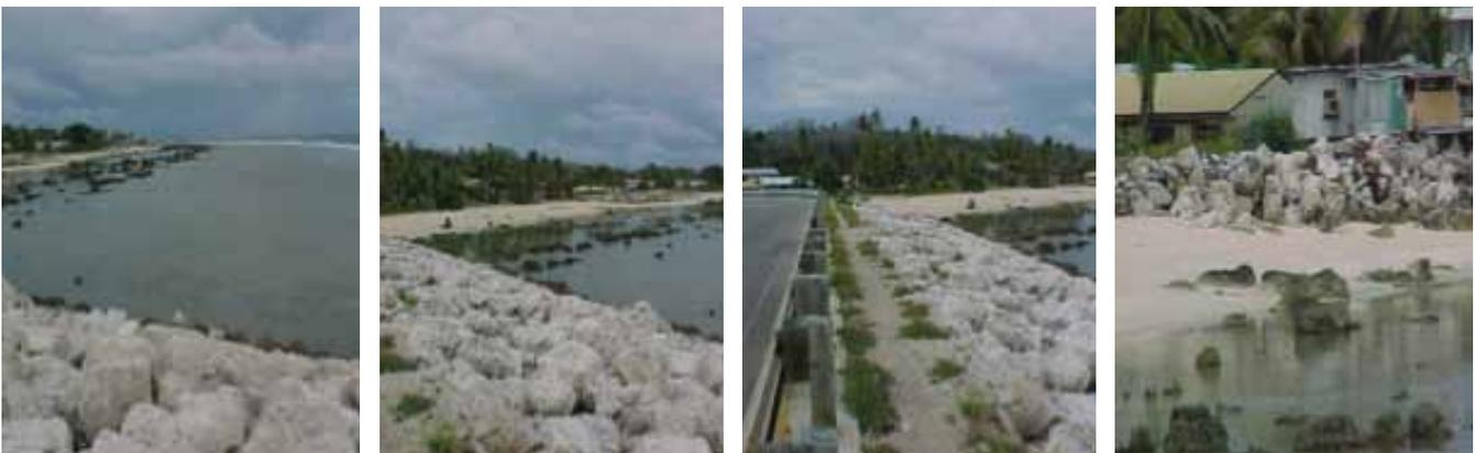
Figure 106 rock revetment. Figure 107 layout of rock revetment. Figure 108 rock wall. Figure 109 rock wall protects a house (Source: Fig.106 - 109: Maharaj, 2000)
