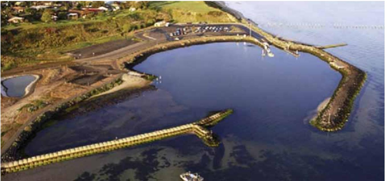
Figure 24: Geotextile Sand-filled Container (Elcorock) Breakwater Example
