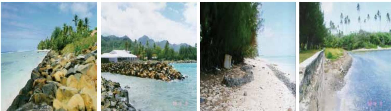
Figure 25 Rock riprap wall, Figure 26 Avarua rock groynes, Figure 27 Gabion basket wall, Figure 28 Ngatangia concrete wall
