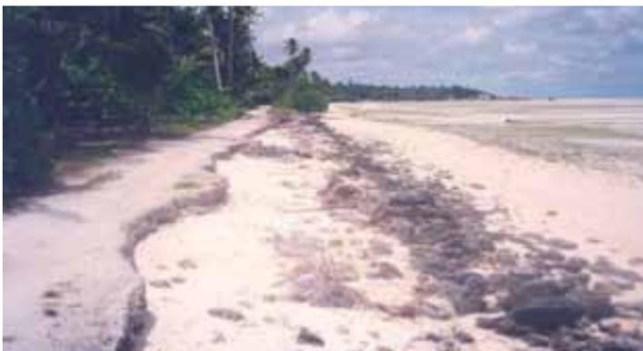
Figure 193 Collapsed seawall in Abemama.
