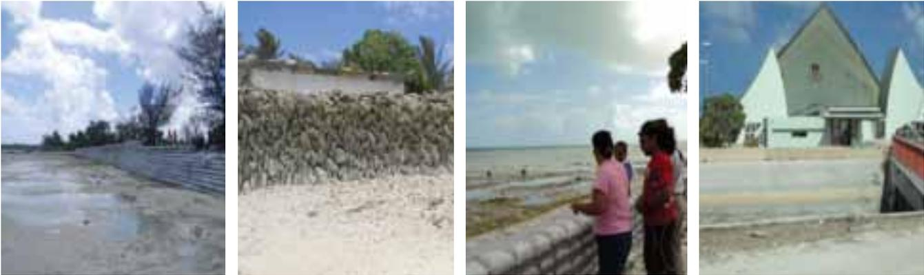
Figure 65 Concrete Sandbag wall. Figure 66 Rock wall. Figure 67 Causeway Concrete wall. Figure 68 Concrete revetment wall at Parliament House.
