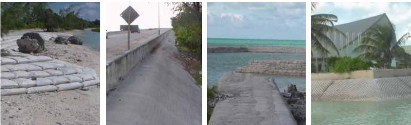
Figure 73 Mangroves and sand bags wall at Bonriki. Figure 74 Dainippon Causeway Bairiki to Betio. Figure 75 Private land-reclaiming project using sand bags wall at Bairiki. Figure 76 Sloping cement wall protecting Parliament House.
