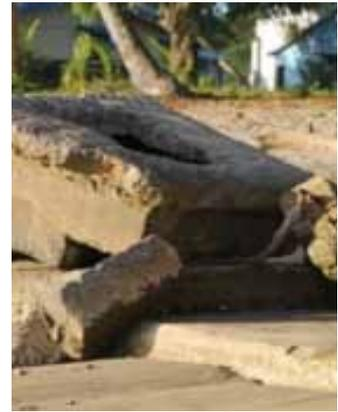
Figure 179 Part of seawall at Lomeri High School collapsed. Figure 180 Same seawall looking from seaside. Figure 181 Poor engineering work
