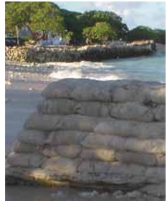
Figure 198 Erosion begins where wall ends. Figure 199 Erosion at end of seawall. Figure 200 Erosion seen at toe of sandbag wall.
