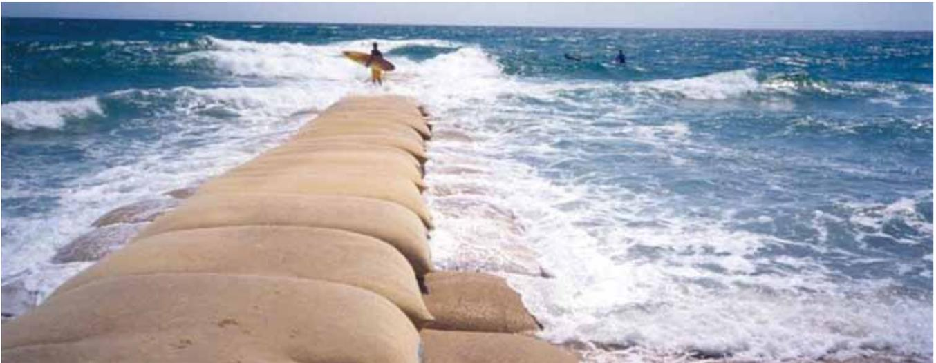
Figure 21: Geotextile Sand-filled Container (Elcorock) Groyne Example
