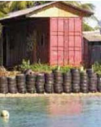
Figure 99 Vehicle tire neatly stacked as seawall.
