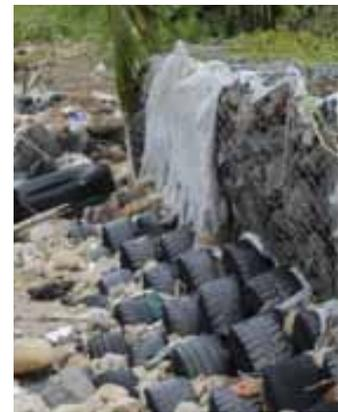
Figure 182 Tire wall collapsed at end of seawall. Figure 183 Tire wall was ineffective. Figure 184 Vehicle tire wall at end collapsed
