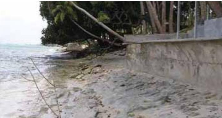
Figure 97 Seawall placed on rock.
