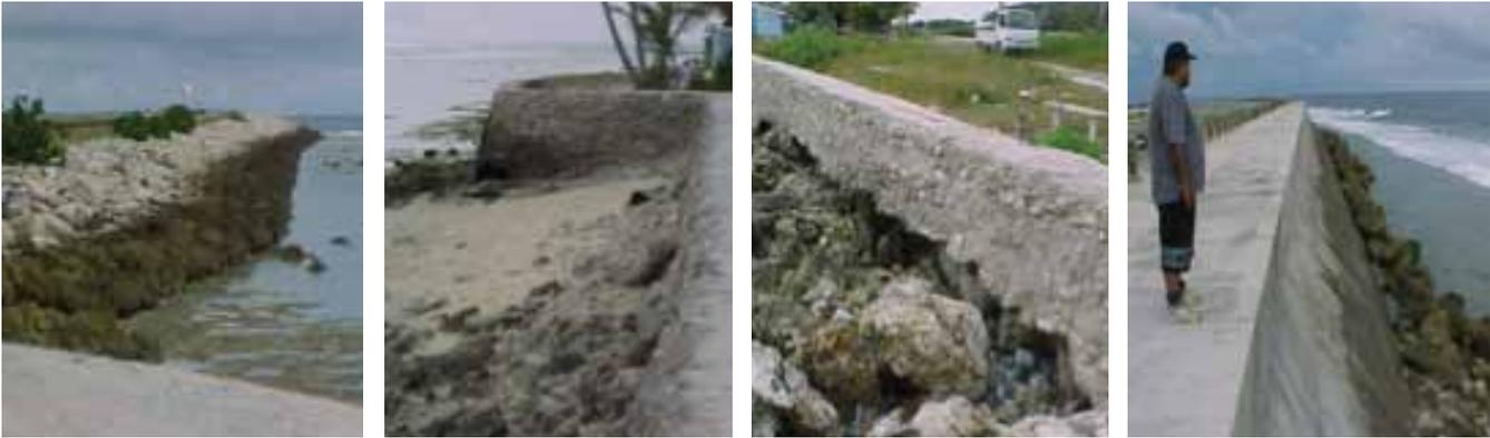
Figure 102 Rip rap rock revetment. Figure 103 Concrete wall. Figure 104 Long concrete wall. Figure 105 Concrete wall with rocks at base-ment. (Source: Fig.102 - 105: Maharaj, 2000).
