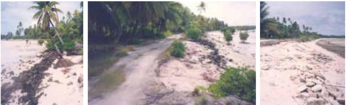
Figure 190 Collapsed wall at Rotima, Nonouti. Figure 191 Eroded road and seawall collapsed at Rotima..Figure 192 Collapsed concrete filled sandbag wall at Nonouti. (Source: Fig.190 -192: Gillie, 1993).
