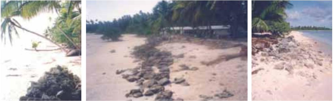
Figure 187 Erosion at end of seawall-Eita, Tabiteuea North. Figure 188 Collapsed seawall-Tewai school, Tabiteuea South. Figure 189 Collapsed seawall at Temotu island, Nonuti. (Source: Fig. 187 -189: Gillie, 1993).
