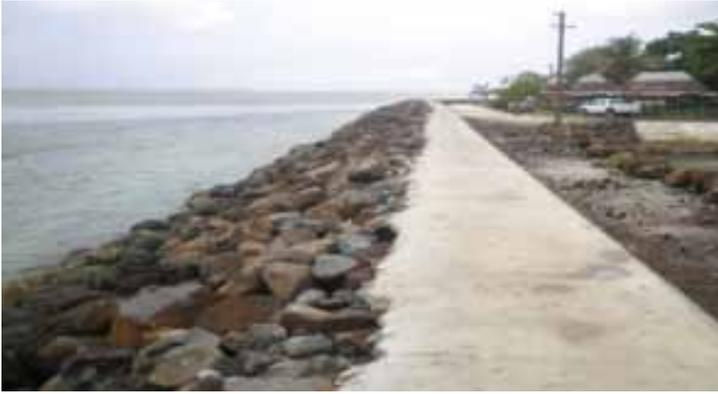
Figure 137 Partial concrete revetment at Piula.
