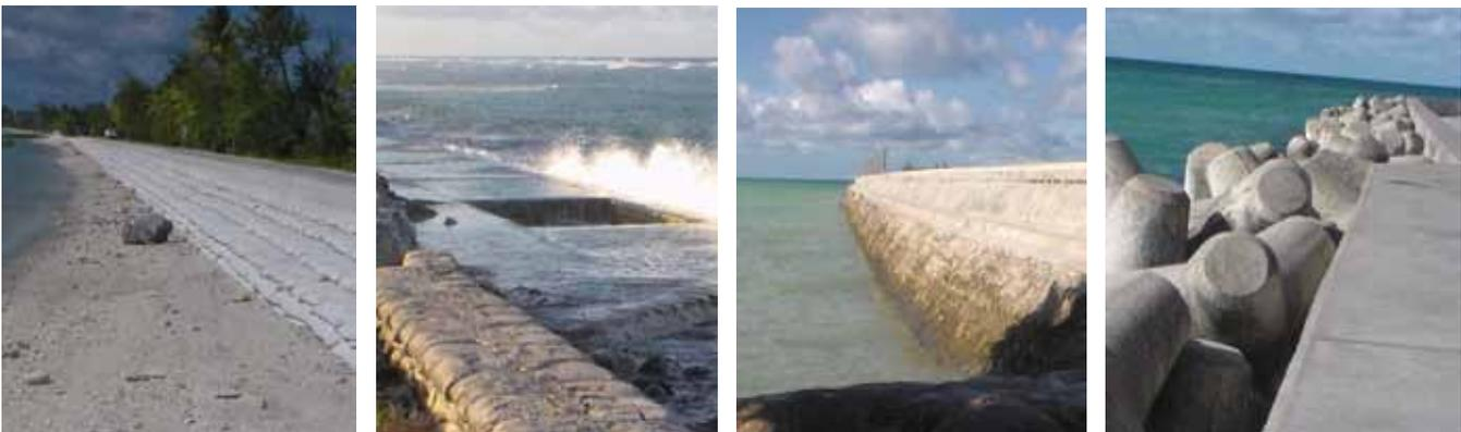
Figure 69 Bonriki Sloping sandbag wall. Figure 70 Concrete slabs at Oceanside of Bonriki airport. Figure 71 Sloping concrete wall at Red Beach, Betio. Figure 72 Wave Breakers at Betio Wharf.
