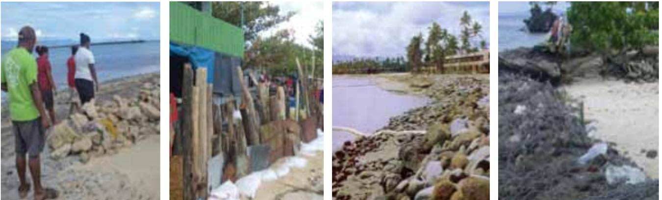
Figure 133 Stone wall at Mou Kele village. Figure 134 Sandbag and tree trunk wall. Figure 135 Rock wall at Gilibwa village. Figure 136 Gabion Basket wall at Los Negros Island.
