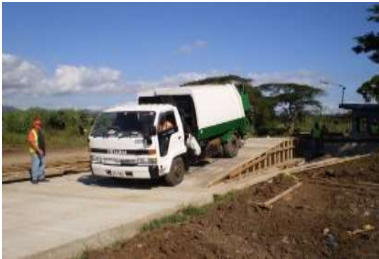
Photo 2: Testing of ramp gradient
