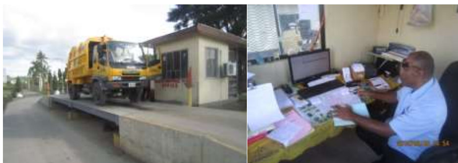
Installed electronic system at Lautoka, Fiji
