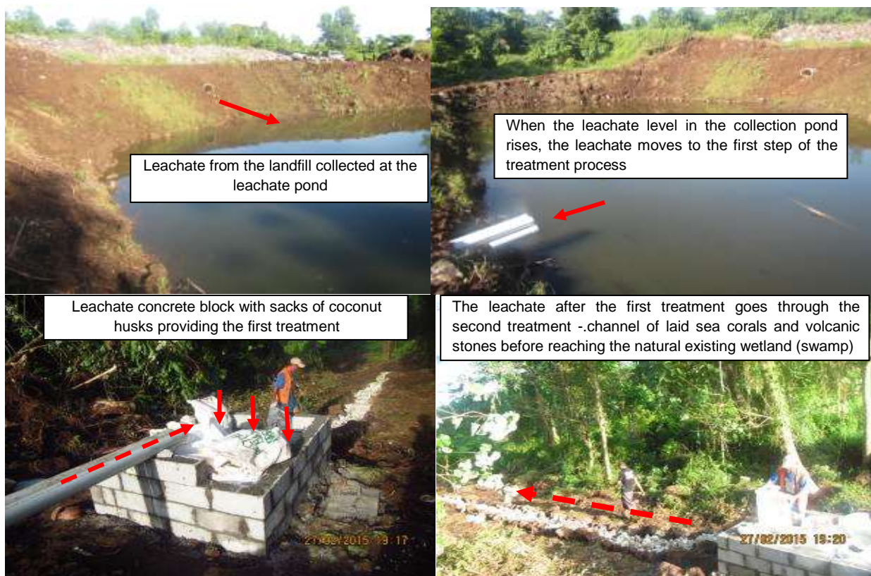
The leachate treatment at the Vaiaata Waste Landfill, Samoa
