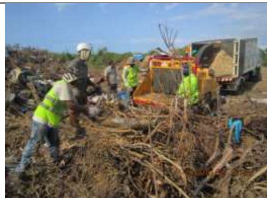
Photo showing chipping of hurricane waste
