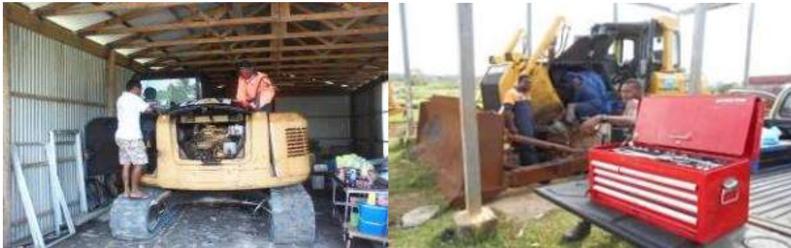
Operators and mechanics doing the regular maintenance in Funafuti (left) and Port Vila (right)
