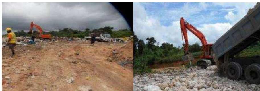
Examples of good daily control of disposal operations at the working face
