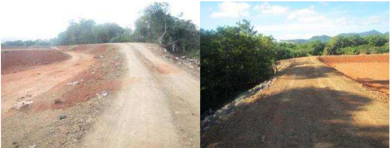
The new road located on top of the embankment
