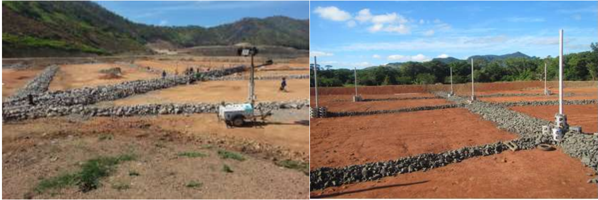
Completed Waste Landfill at Baruni, PNG (left) & Labasa, Fiji (right)
