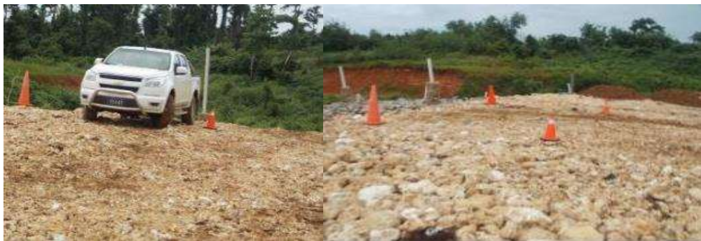
Example of daily working face preparations to guide disposal operations
