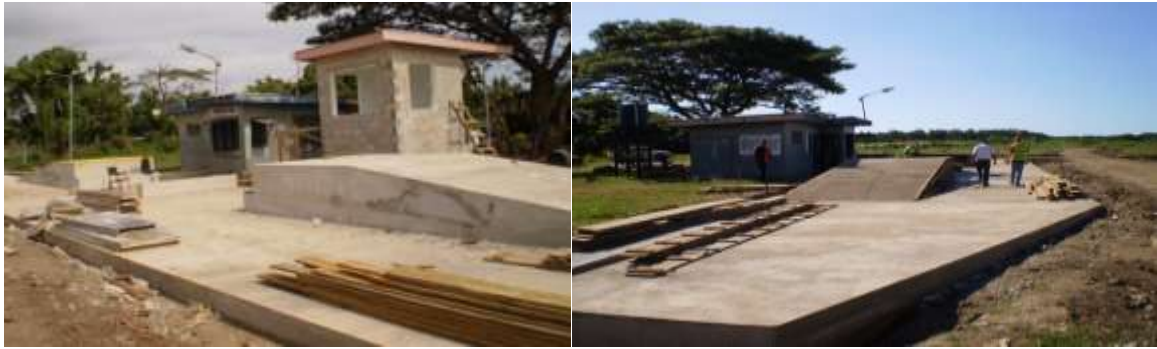
Photo 1: Weighbridge Construction Works. Constructed above ground due to flood-prone area
