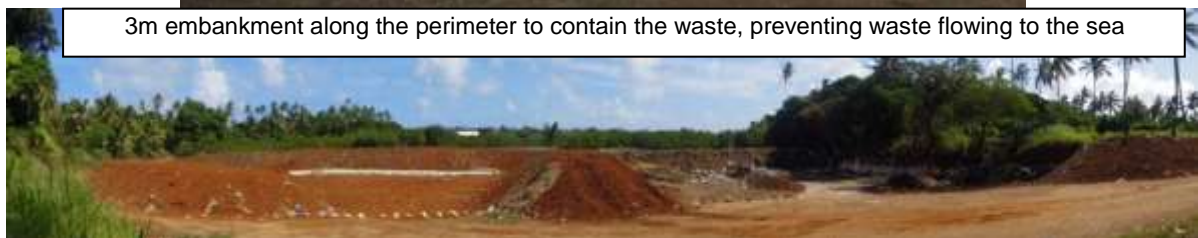
After improvement works
