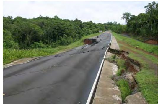
Figure 7 Collapsed national highway in Ngchesar State after heavy rains in 2009
